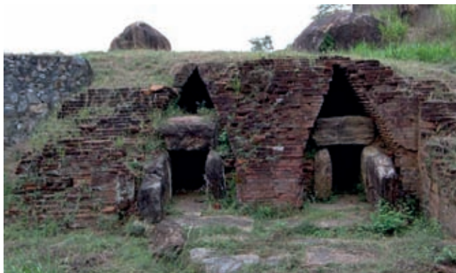
Figure 15.38 - An ancient tank bund
